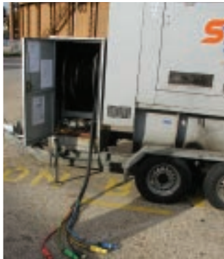
Reliable connections for field installation power distribution systems such as mobile generators.
