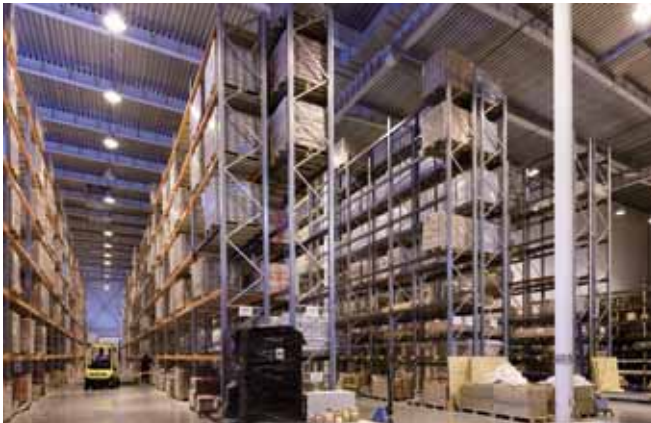
High bay lighting
